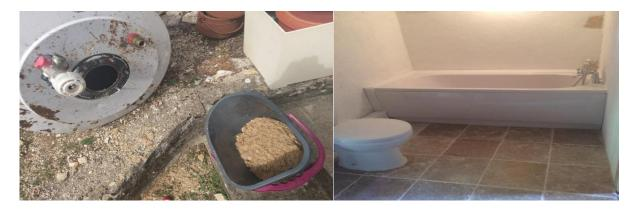
Limescale can seriously damage or impair the operation of plumbing and its various components. (Bucket in photo, is full of limescale from a defunct 14 year old hot water tank.) I can provide a free quote/ devis and advise on possible solutions for your limescale or any other issues you may have.
